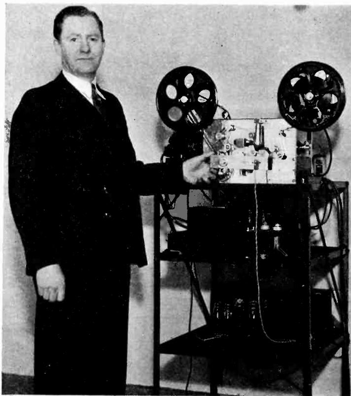
J. A. Miller with his sound-track engraving apparatus. The magnetically controlled cutting stylus is mounted beneath the film in the topmost section. Recording and play-back amplifiers are shown below
