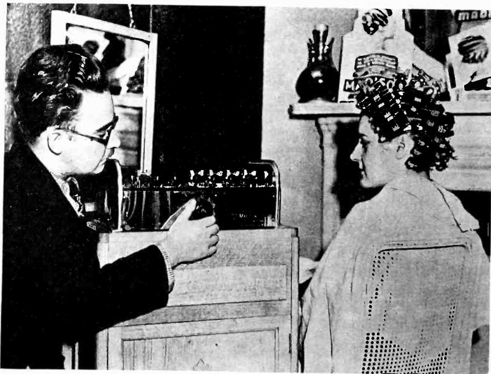
With the aid of electrically-conducting curlers, and in the presence of a high-frequency field, this "permanent-wave" machine in a London beauty-shop avoids heavy wires to operate the heaters
